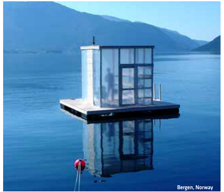
5.B Floating pontoon
