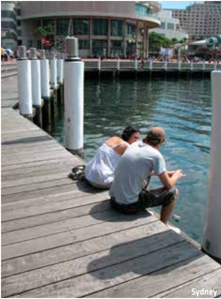
2.J Wooden jetty
